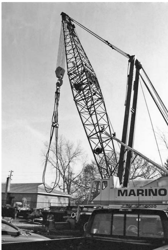
FIGURE 25.2 Rigging sling attached to crane's hook.
