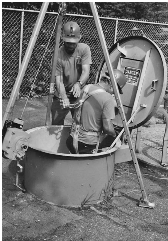
FIGURE 25.4 Confined space entry.
