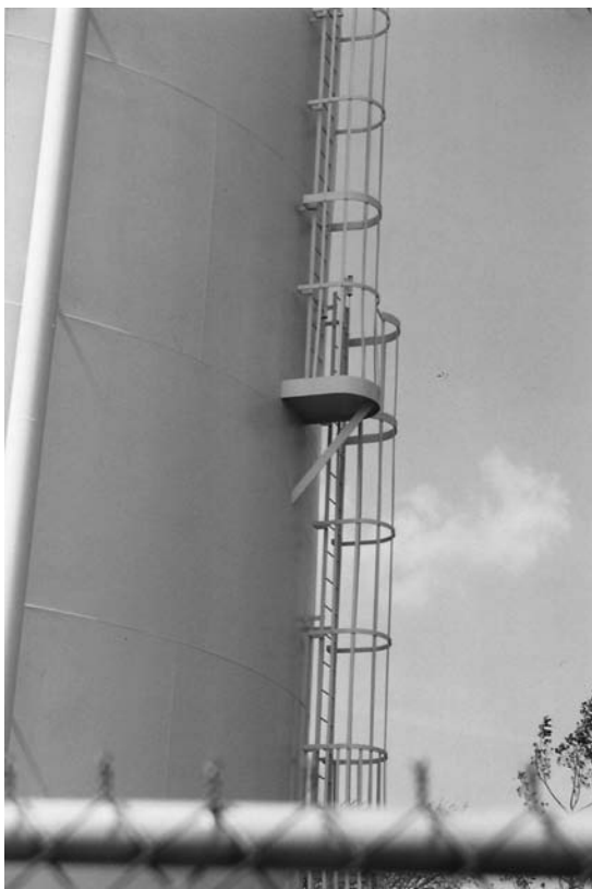
FIGURE 25.17 An example of a fixed ladder.
