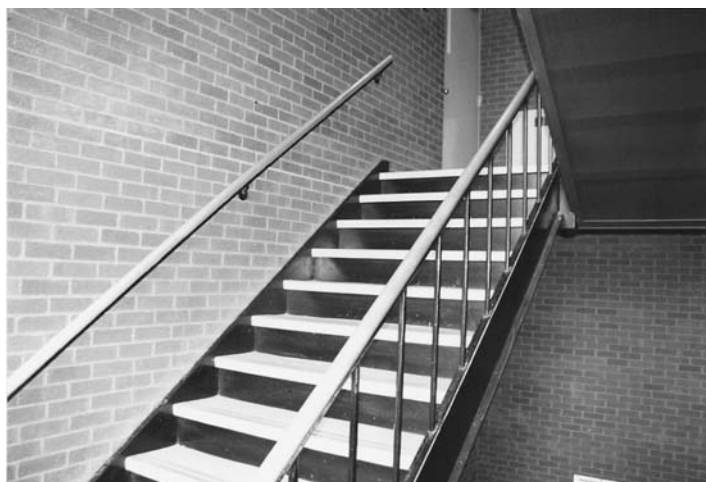
FIGURE 25.21 Example of a stair rail and handrail.
